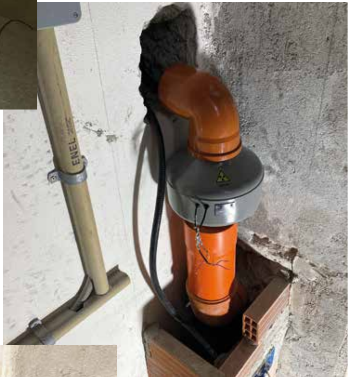
SICURBOX control unit installation for control, monitoring and management.
